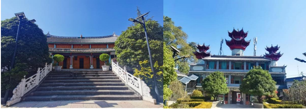
Figure 4. Mosque of Shangxingzhuang Village
