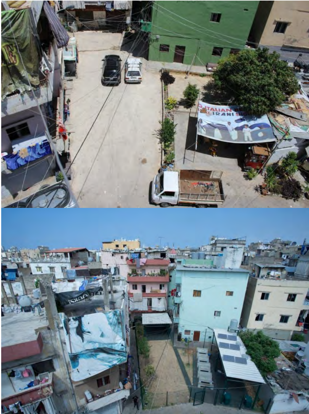
Figure 3: Location of the lot before and after the public space implementation
