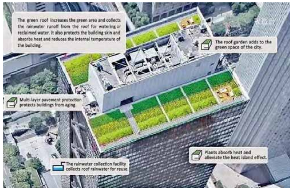
Figure 12. Green roofs of the buildings
