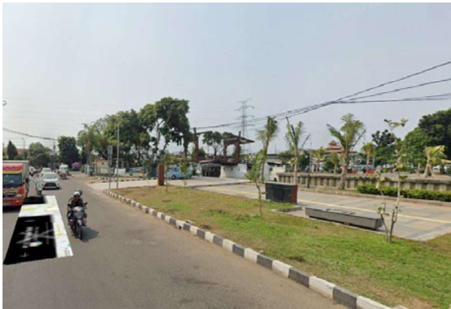
Figure 4 : Kali Besar today in Jakarta, 2024, Google street view.
