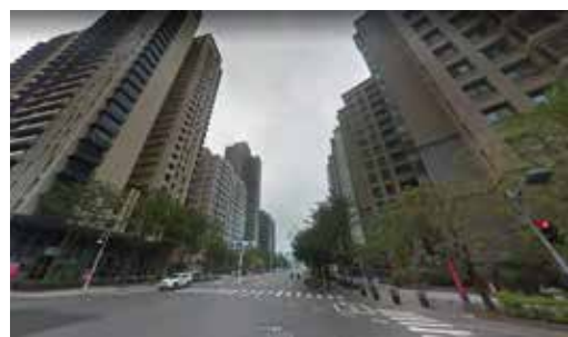
Figure 12 The northwest side of the study area
