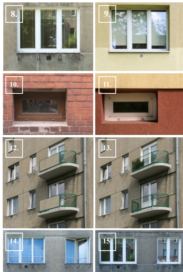
Figures 8. – 15. Examples of original (left) and secondary (right) design solutions from ZUS modernism housing estate in Lodz, Poland: 8. & 9. colour and pattern of plaster; 10. & 11. plinths; 12. & 13. balconies; 14. & 15. windows' subdivides. Source: Jakub Zasina (2013).
