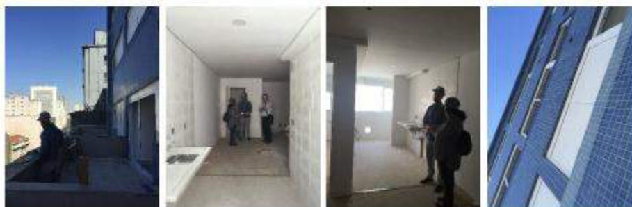
Figures 10-13 – Ipiranga Building – Renovation Work (Camila D'Ottaviano 2016)
