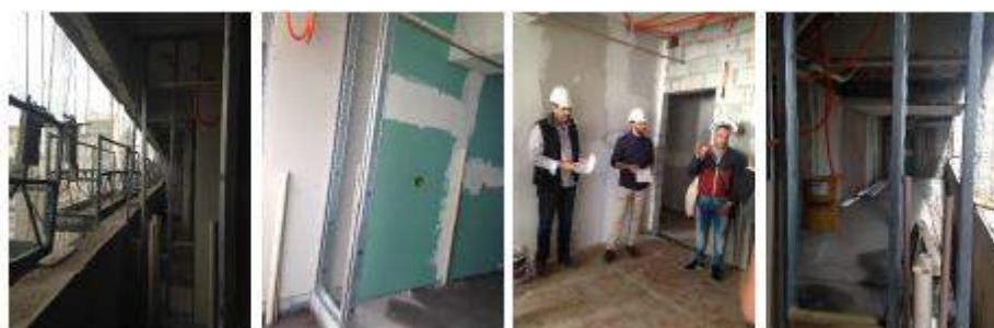
Figures 4-7 – Ipiranga Building – Renovation Work
