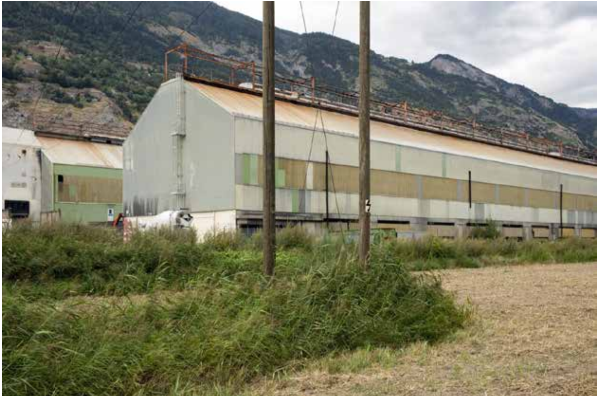
Figure 16 – The former electrolysis halls. (copyright: Marcello Modica)
