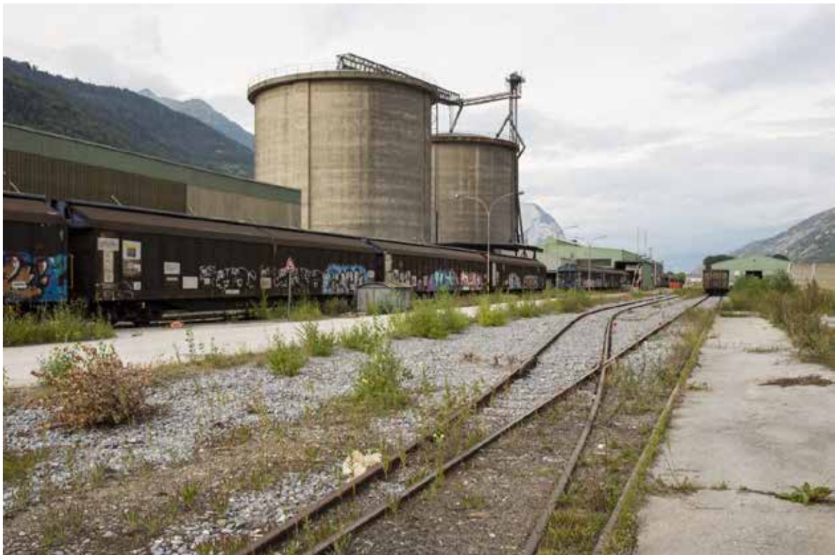
Figure 17 – The site internal railway yard and the two alumina silos in the background. (copyright: Marcello Modica)
