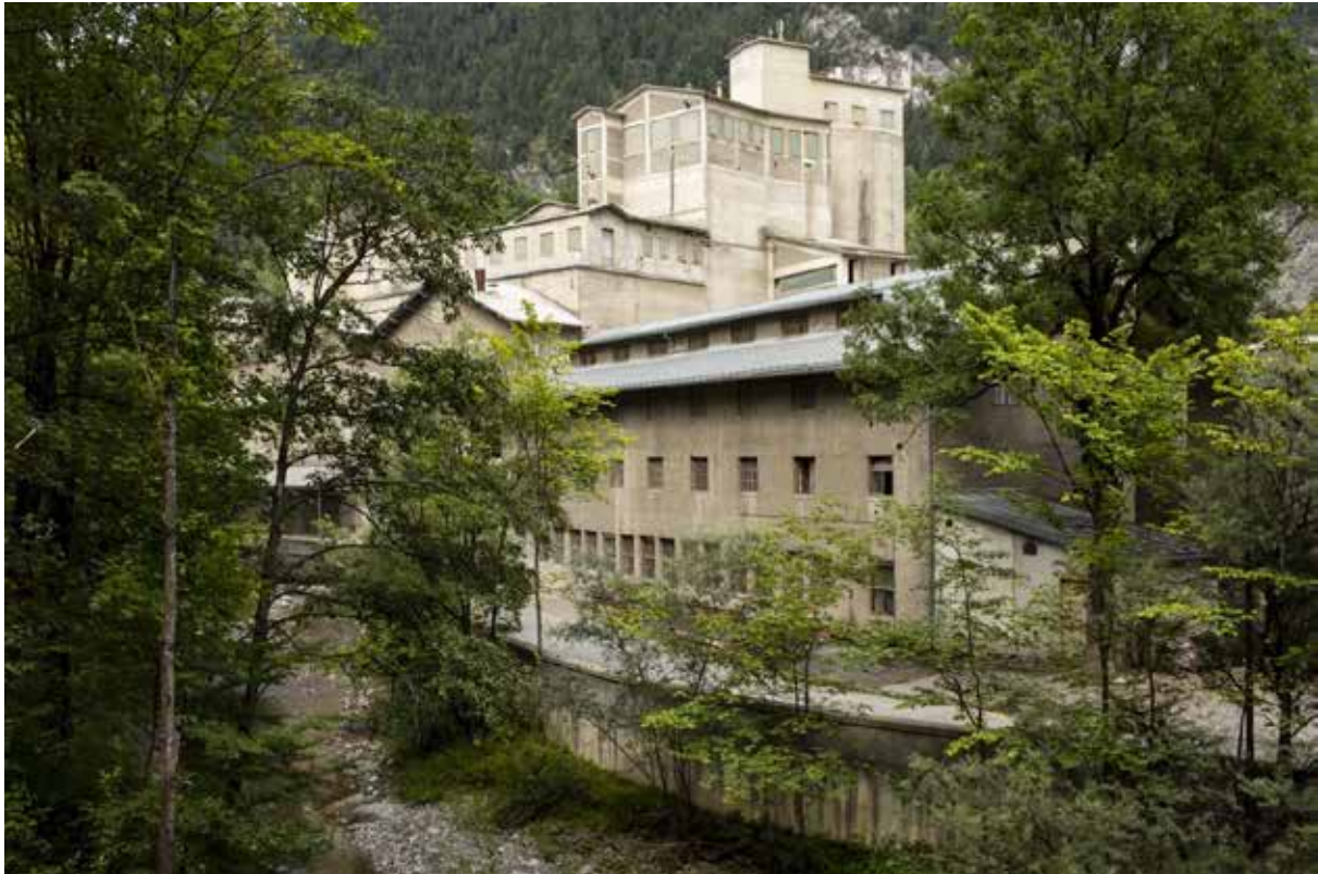
Figure 4 – The Eiberg cement plant along the rectified Weißache (copyright: Marcello Modica)
