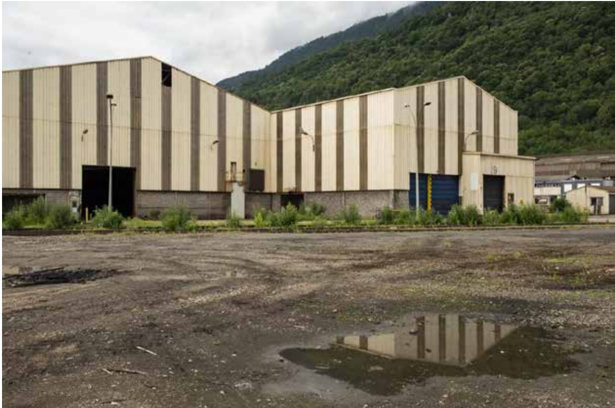
Figure 8 – The former rolling mill halls surrounded by leftover open spaces (copyright: Marcello Modica)
