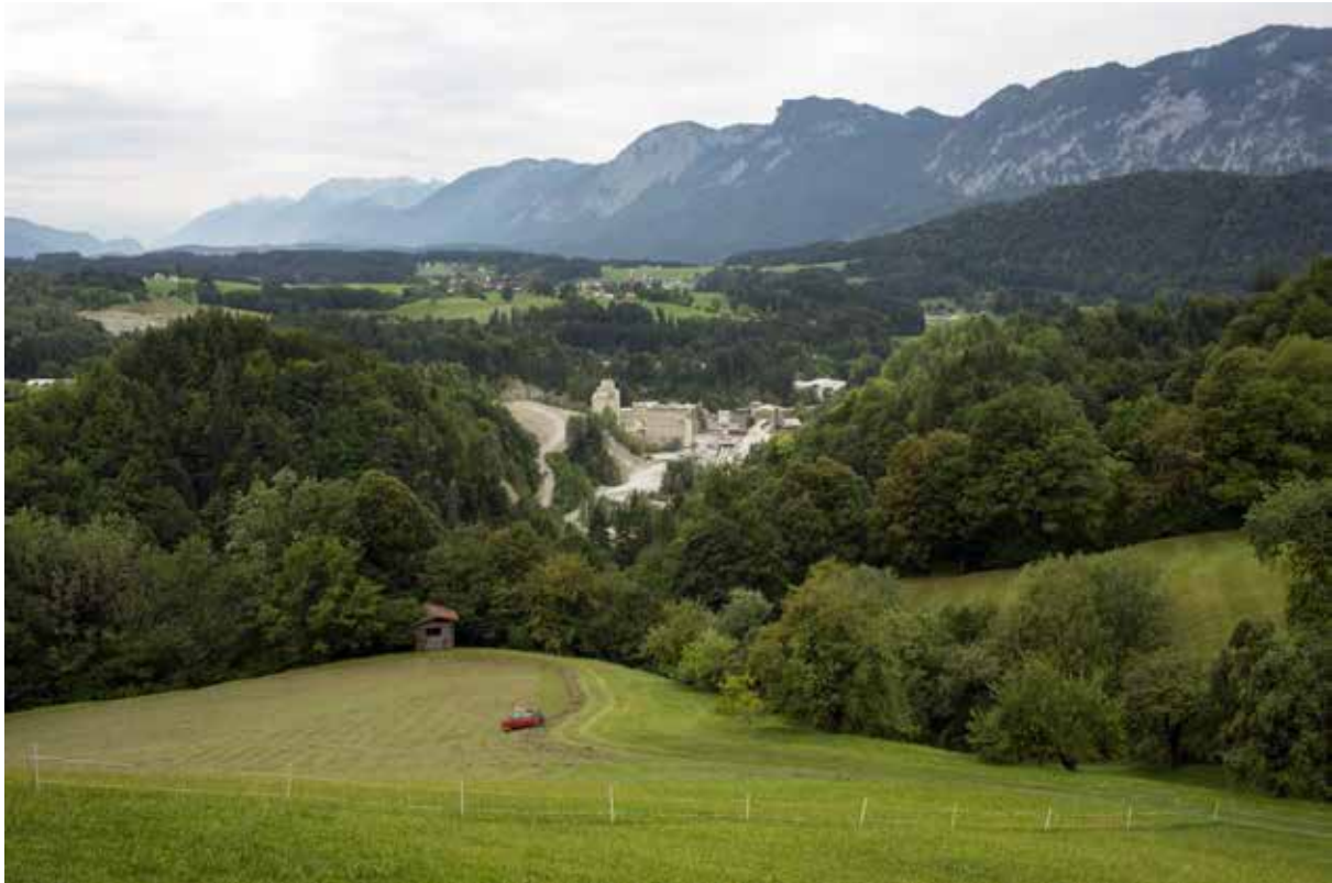
Figure 3 – Overview of the Eiberg cement plant from the Pölven foothills (copyright: Marcello Modica)
