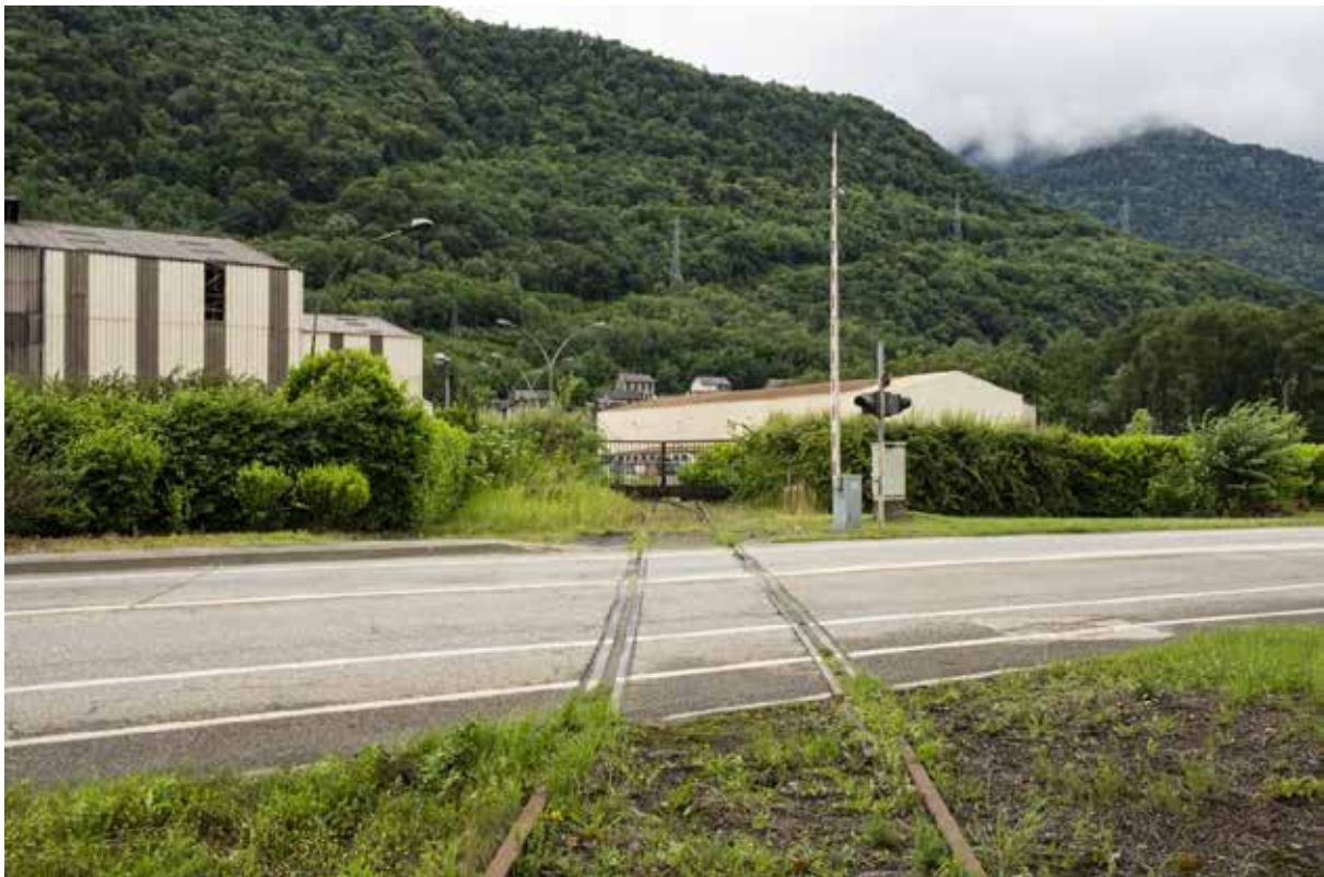
Figure 9 – One of the railway links between the site and the Grenoble-Chambery regional railway (copyright: Marcello Modica)
