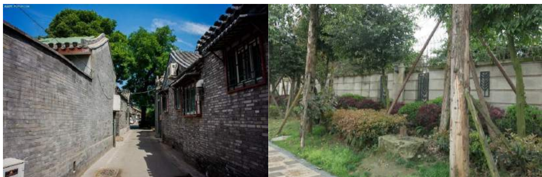
Figure 4 –Wall in “Hutong” (Author, 2015) | Figure 6 –Wall of “Cheng Nan Yi Jia” in Chengdu (Author, 2017)
