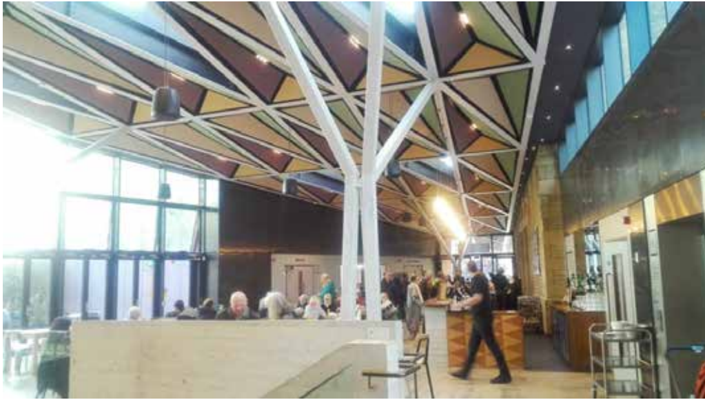
Figure 9 New hall of Square Chapel Arts Centre, view from the renovated upper floor of Bradley Hall
