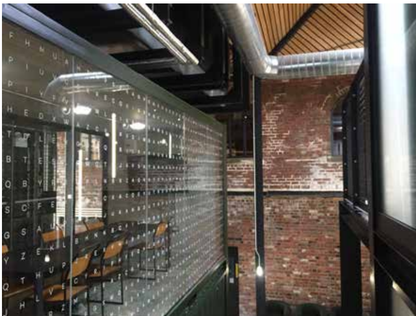
Figure 5 Adaptively reuse of recycled shipping containers as plug-in meeting spaces of the red-brick shell
