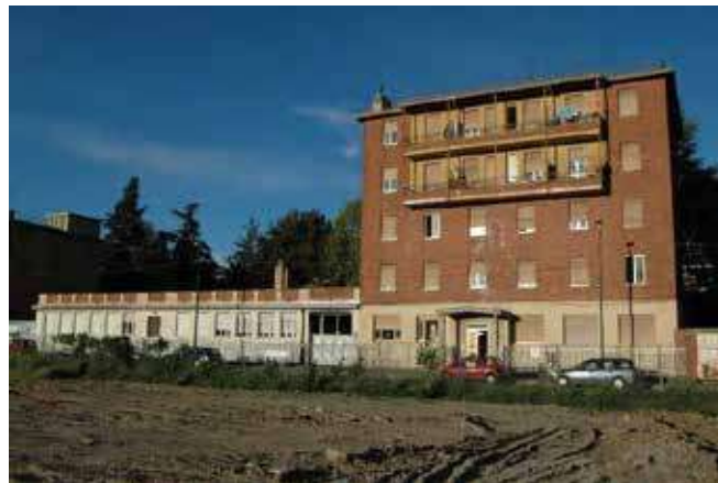
Figure 1 View of the building from via Madonna de la Salette, before the intervention.
