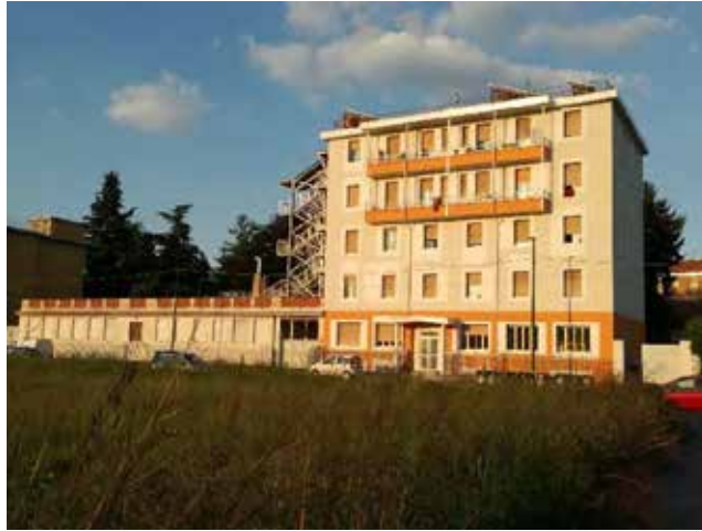
Figure 2 View of the building from via Madonna de la Salette, after the intervention.
