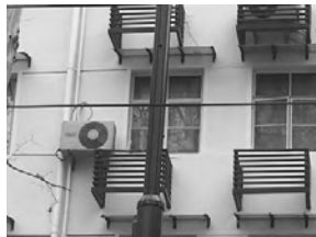
Figure 10 Air-conditioned External Aircraft that not Suspended in Required Position (Source: Author's self-photograph)
