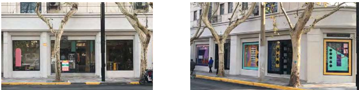
Figure 16: Fiu2 Gallery Facade Restoration (Source: Author's self-photography)
