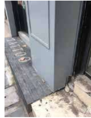
Figure 7 Renovation Details (2) (Source: Author's self-photography)
