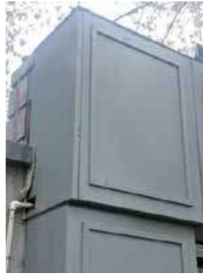
Figure 6 Renovation details (1) (Source: Author's self-photography)
