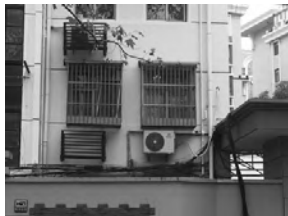
Figure 10 Air-conditioned External Aircraft that not Suspended in Required Position (Source: Author's self-photograph)
