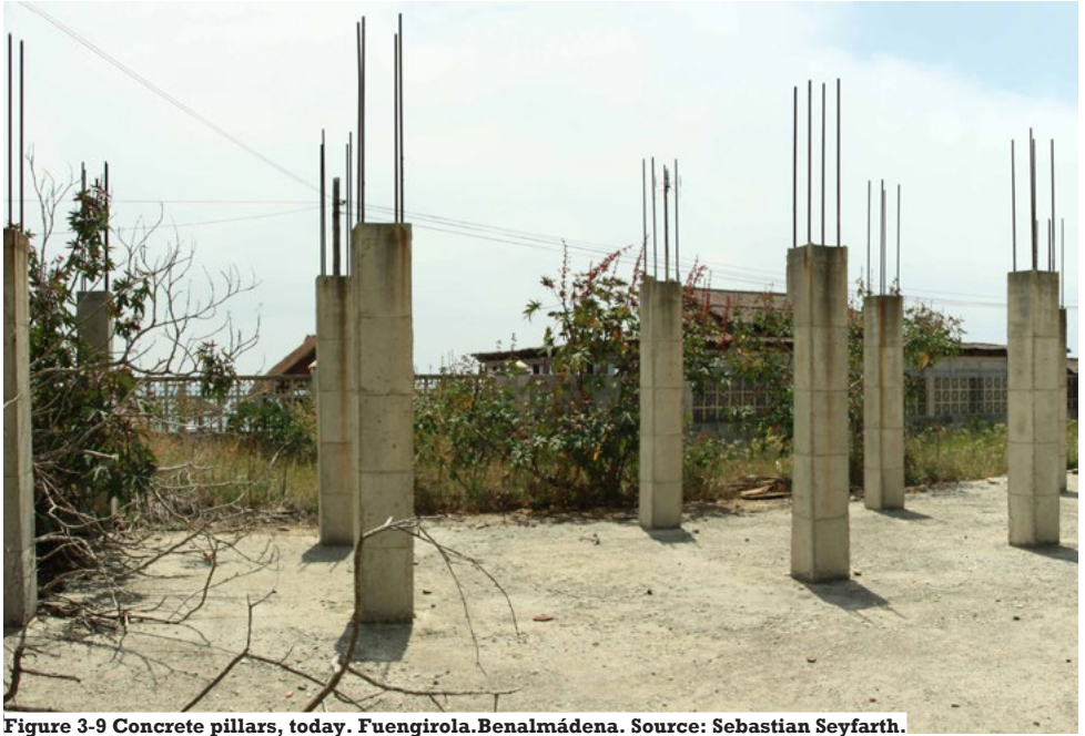
Figure 3-9 Concrete pillars, today. Fuengirola.Benalmádena. Source: Sebastian Seyfarth.
