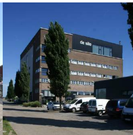
Figure 4 – The retrofitted flour mill (a2o architecten)
