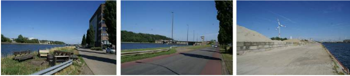
Figure 2 – The Albert Canal between Hasselt (left) and Genk (right).
