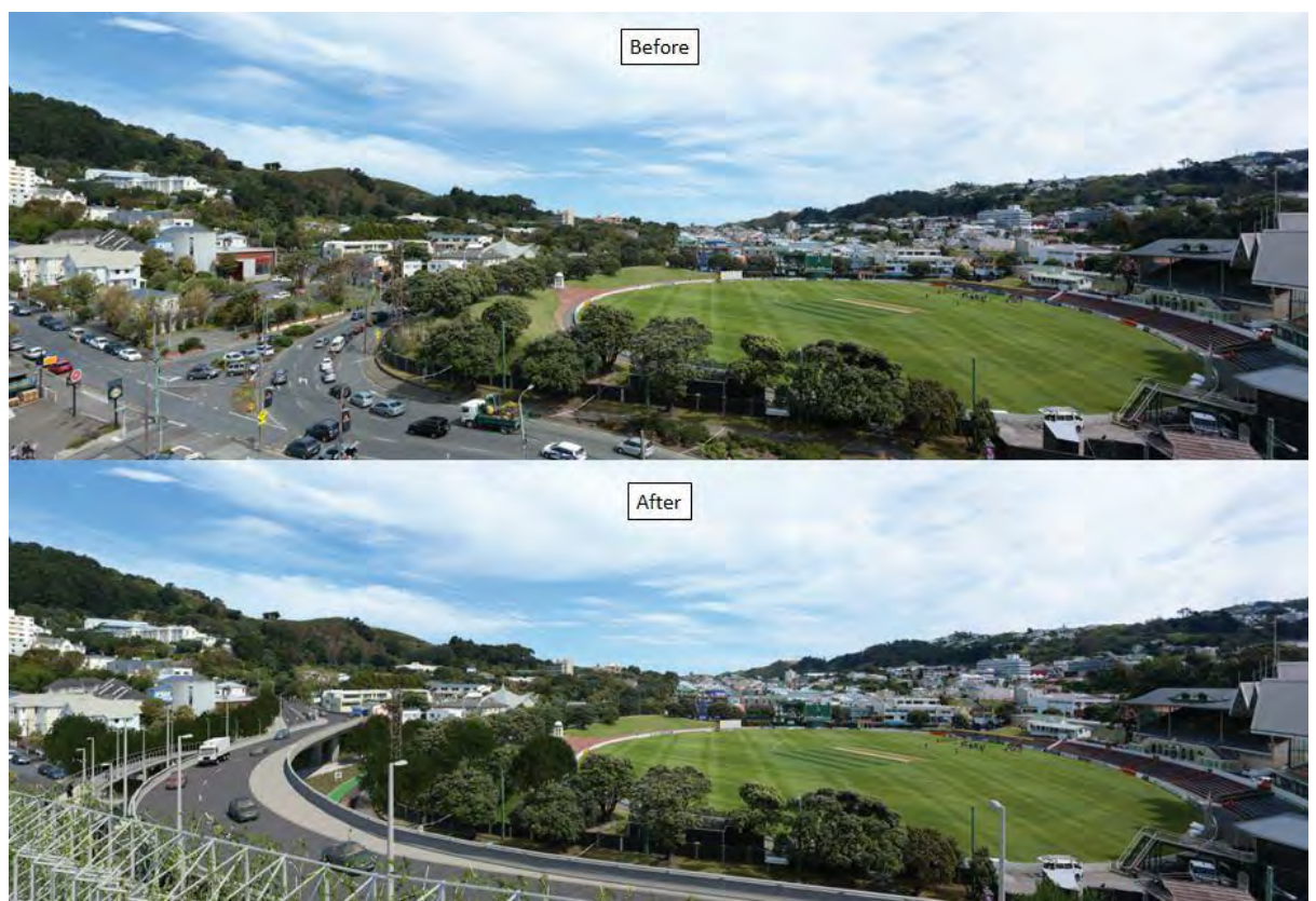
Figure 3 Before and after views of what the Basin Reserve project would look like. Source: http://transportblog.co.nz/2013/11/27/photo-of-the-day-basin-bridge/
