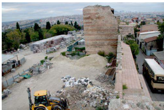
Figure 9) Construction site at the Theodosian Land Walls (source: author, 2015)
