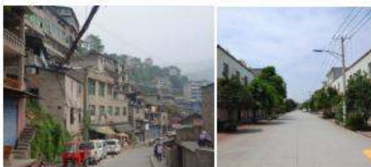
Figure 6 - Small-scale street system in old town of Fengjie County, Chongqing | Figure 7 - Big-scale street system in Caichang County, Chengdu
