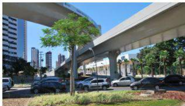
Figure 8 - Viaducts in operation after construction. Photo accessed at: http://tribunadoceara.uol.com.br/noticias/cotidiano-2/manifestantes-relembrem-momentos-de-luta-dois-anos-apos-ocupacao-do-coco/attachment/dsc_8396/ .
