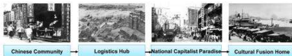
Figure 4 -Historical Pictures in 1990-1930 Source: Research on Conceptual Planning of Shanghai Fuxing Dock Land
