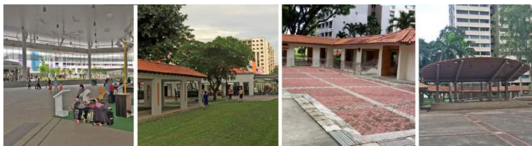
Figure 7 - Examples of categories of neighbourhood spaces: (from left to right) Category A - Bedok Town Square, sheltered plaza next to the subway station and a shopping mall; Category B - Space adjacent to food court, badminton court and a green open space in Woodlands; Category C - Paved open space between the housing blocks in Woodlands, next to a frequently used covered walkway; and Category D – An empty underused amphitheatre in Bedok
