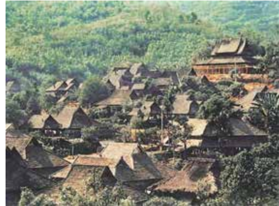
Figure 6. Aerial View of Jinghong Dai Village in Yunnan Province, China (SUN Dazhang, 2004)
