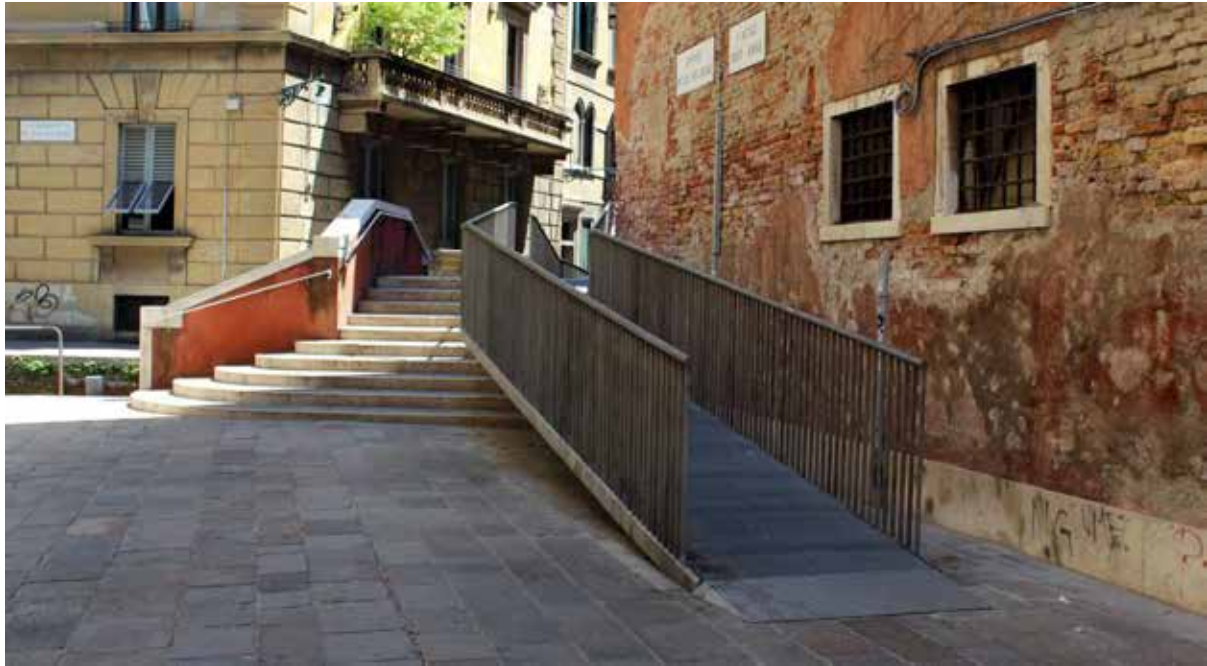
Figure 6. Ponte delle Sechere, an example of a fully accessible bridge. In this case the bridge has been equipped with both handrail on its brick wall (left) and a facilitated step ramp.
