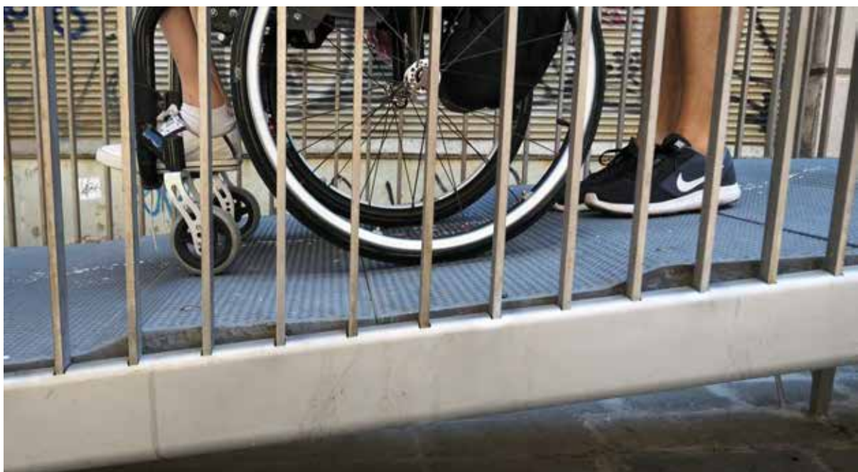
Figure 7. Example of facilitated step made up of two units (gradient 14% - 6%) and a triangular chamfer (gradient about 42%). Average step gradient is 13.4%.
