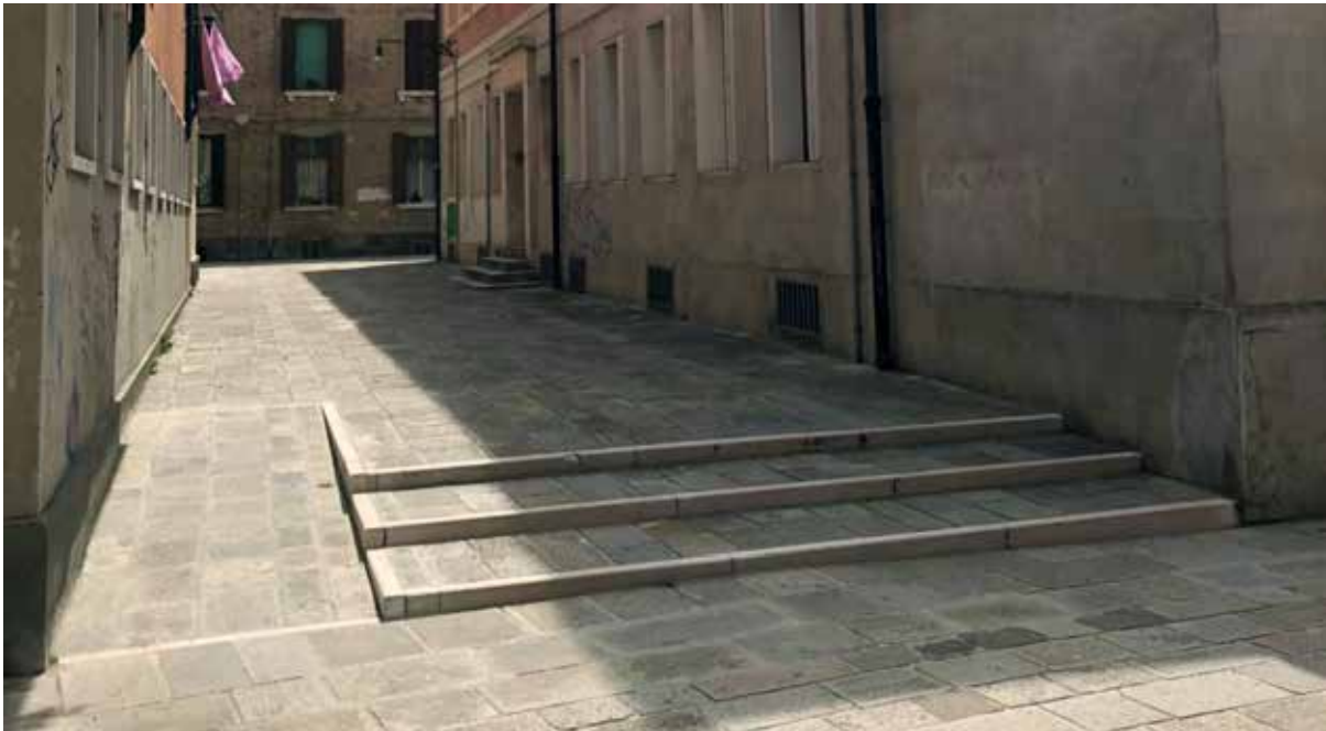
Figure 8. Ramp with a gradient of 5% to get over a pavement height difference between two alleyways.
