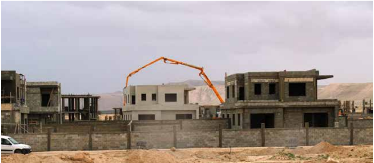
Figure 7: Residential Villas construction in phase Two, Source: Mohammed Isayed, 2019
