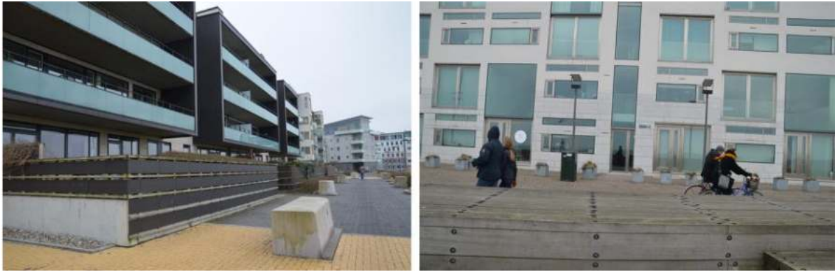
Figure 8, left: the semi-private interface of Dania Park; right: the solid edge of Promenade
