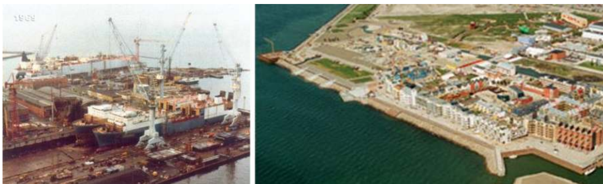
Figure 2, The regeneration of Western Harbour, left 1969, right 2001: Bo01Expo opening
